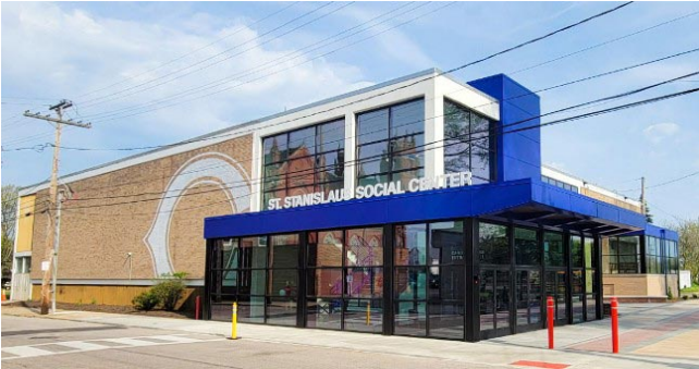
The newly renovated St. Stanislaus Social Center was dedicated on April 28, culminating the yearlong upgrade to the popular Slavic Village venue.
