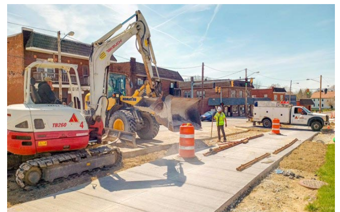
Sidewalk construction along Garfield Blvd. should be completed in the next two weeks, said Allega supervisor Dave DiCillo, at a Ward 3 meeting Monday.
