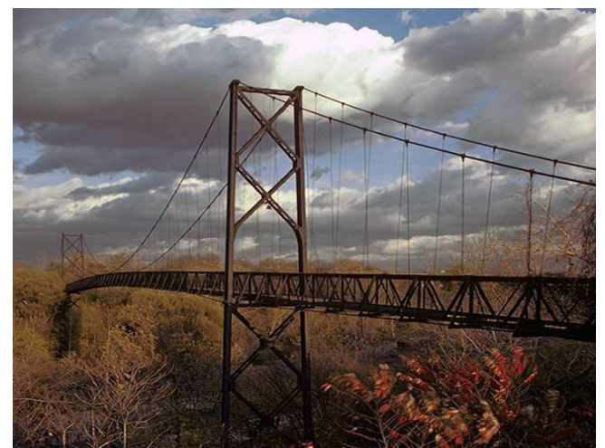
Sidaway Bridge as it looks today. Photo by Tony Brancatelli
