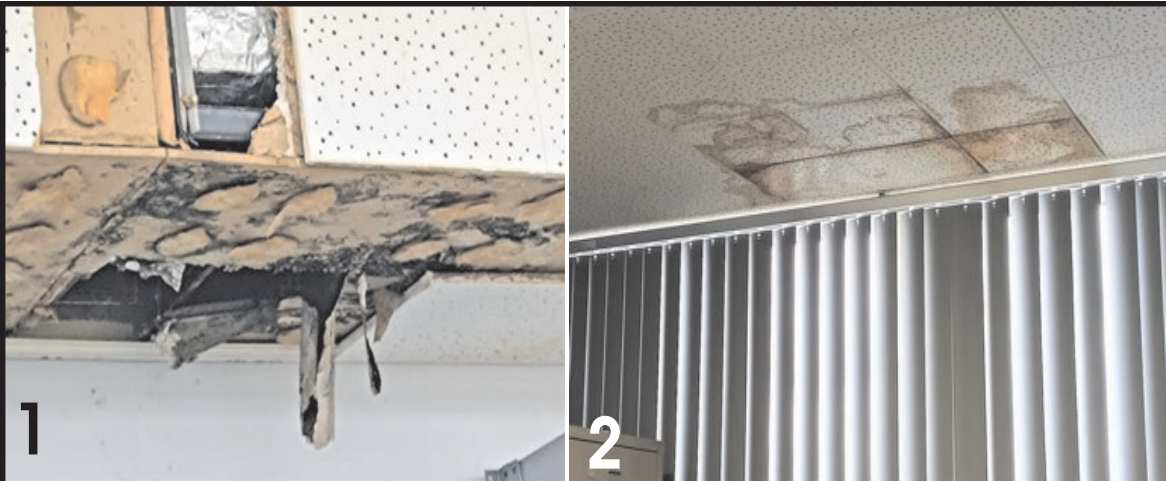
Pic. 1 & 2 - sewage leaks on the ceilings in the locker rooms. Pic. 3 & 4 - corroded pipes in the utility room Pic. 5 - ladies bathroom with a broken stall and leaky ceiling
